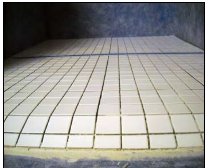
Thin Bed Installation
